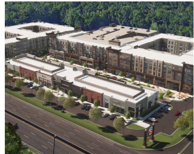
The District at 1515 Parsippany, NJ Construction Retail & Multifamily 498 Units
