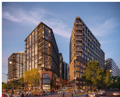
The Stacks Washington, D.C. Construction Mixed Use 1,100,000 SF
