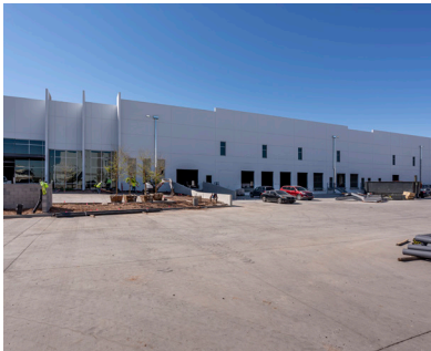
Central Logistics Center Phoenix, AZ Acquisition Industrial 1,138,144 SF
