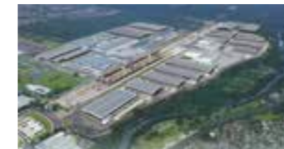
Australia Moorebank Intermodal Terminal , New South Wales
