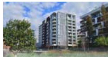
Australia Thornton , Penrith
