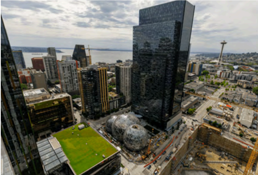
Amazon's Campus in Seattle. Amazon has trialed new retail concepts in the city.
