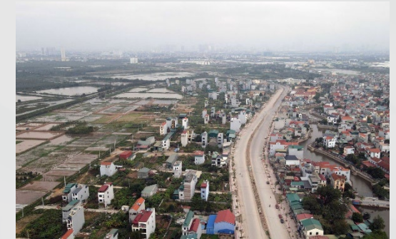
Lai Yen - Van Canh street Exp. To Be Completed: 2024
