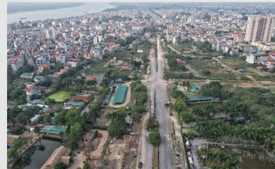
Road connecting Nguyen Van Cu street to the end of resettlement area in Ngoc Thuy ward Exp. To Be Completed: 2024
