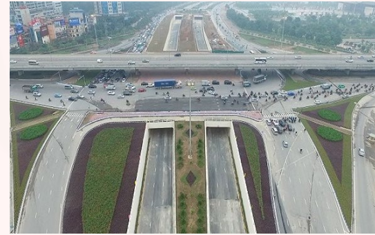
Ring Road 3.5 (Thuong Cat bridge to National Road 32) Exp. Construction: 2026
