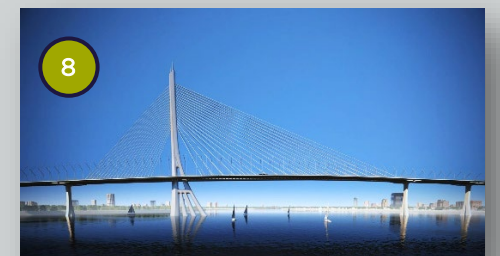
Can Gio Bridge
