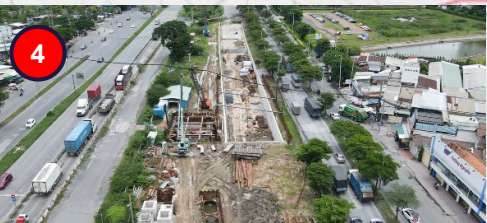
Nguyen Van Linh underground tunnel
