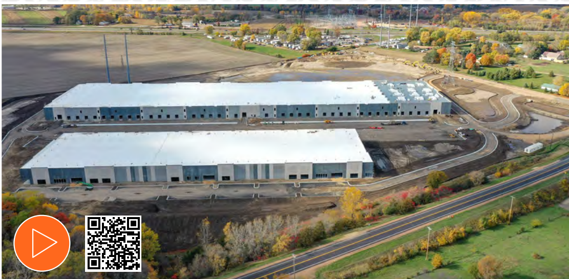
Construction photo, October 2023
