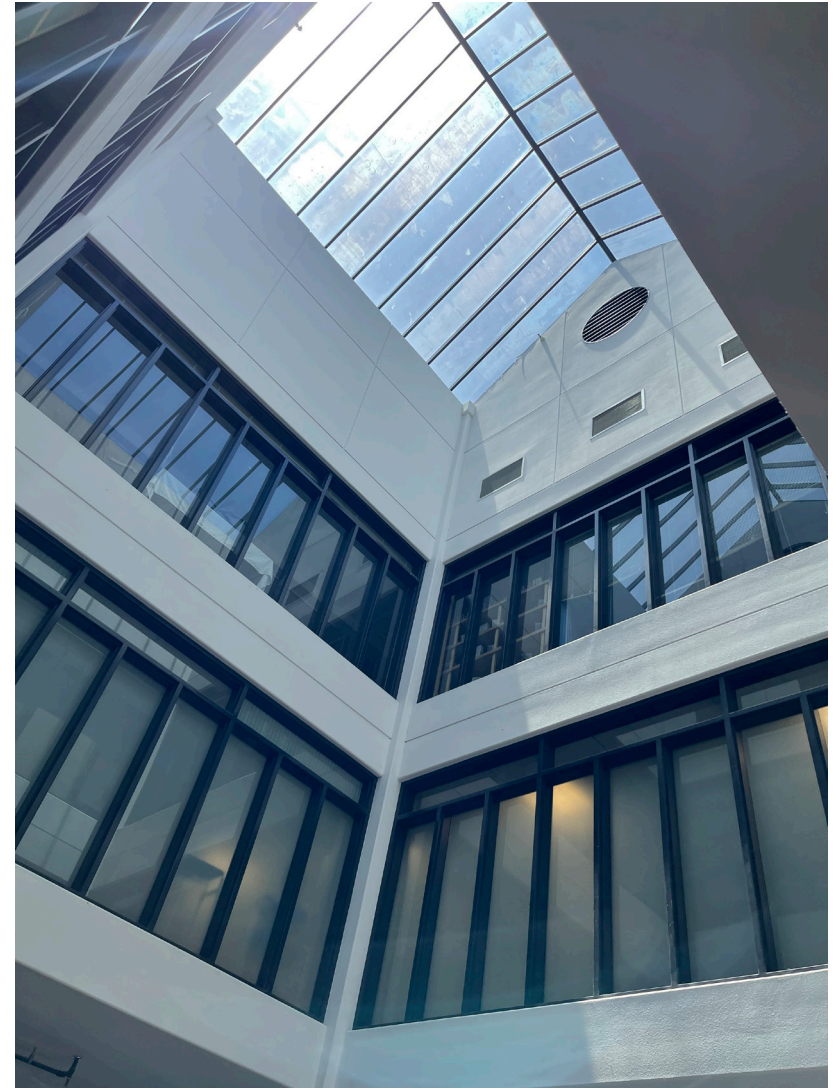
Looking up from Ground Floor
