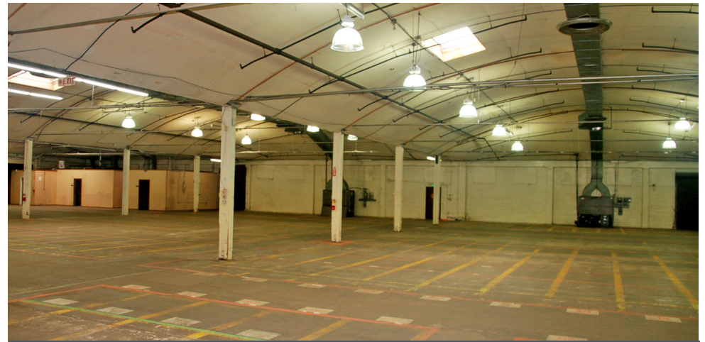
INSULATED, AIR CONDITIONED WAREHOUSE
