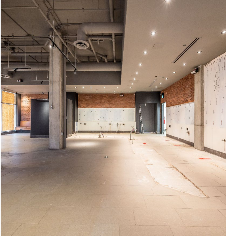
Services in place
