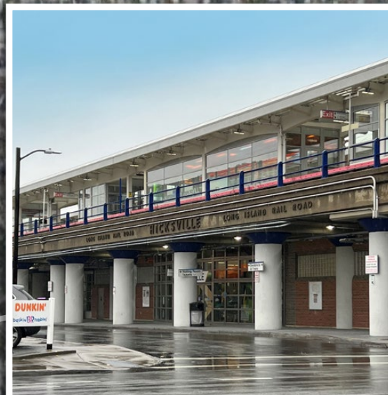
HICKSVILLE LIRR STATION
