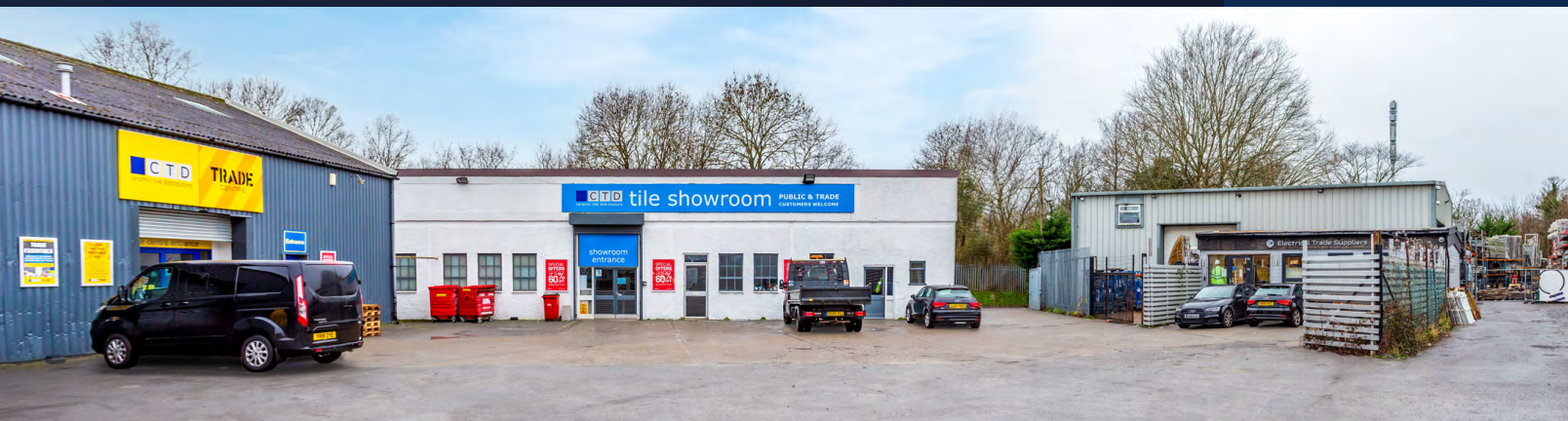
Units C, D & E
