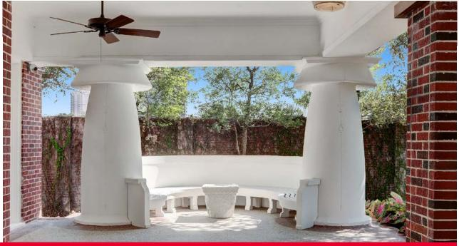
The architectural design of the columns was a "wide-span, reinforced concrete structure bracketed by a cantilevered canopy on the north end and an inglenook on the south, framed by a bulbous concrete column."
