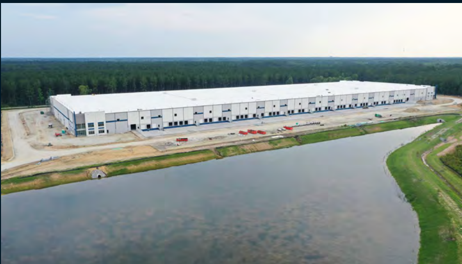
Concrete Truck Court and Drive Aisle
