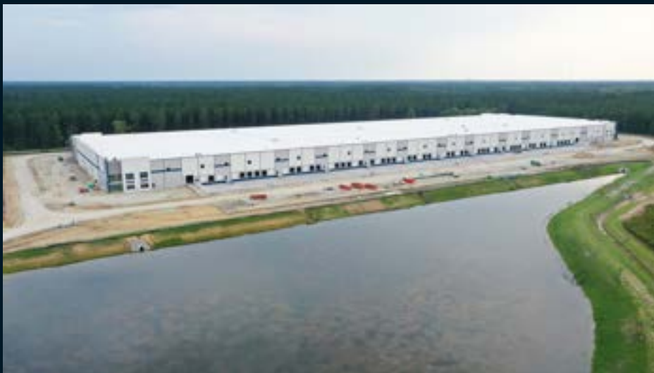
Concrete Truck Court and Drive Aisle
