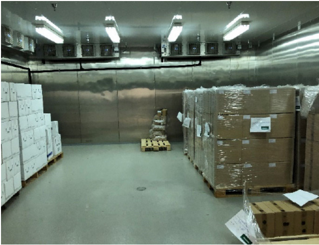
Cold Storage Room
