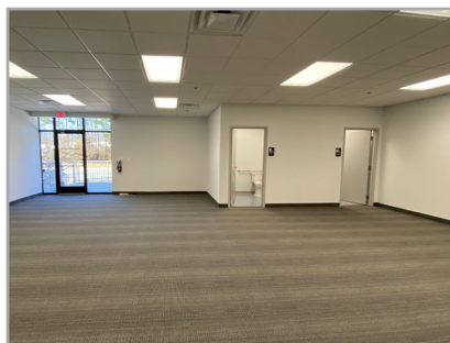
Newly Constructed Office Areas
