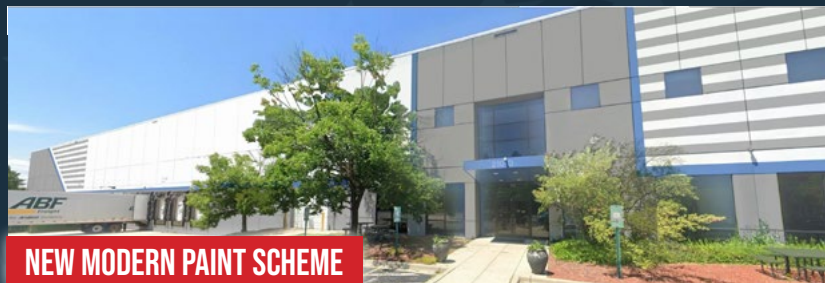
NEW MODERN PAINT SCHEME
