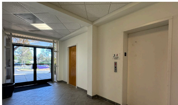
Elevator Lobby & Office Entrance
