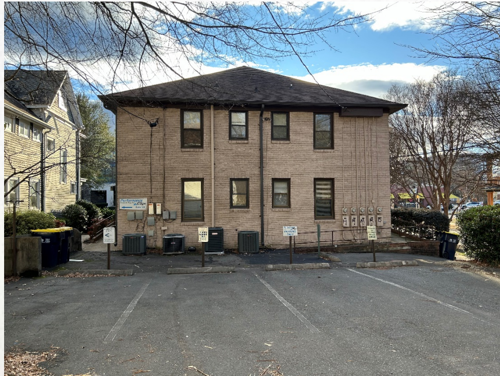
BACK OF OFFICE AND PARKING LOT
