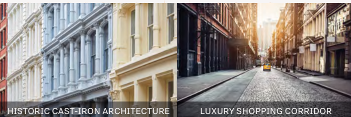
HISTORIC CAST-IRON ARCHITECTURE
