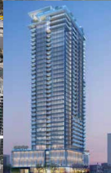
TRAMMEL CROW BUILDING UNDER CONSTRUCTION
