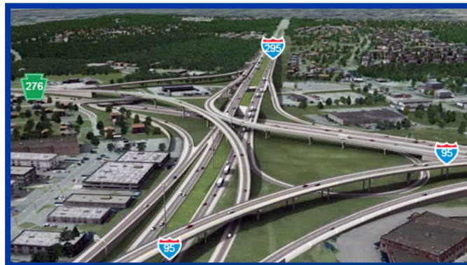
PA Turnpike / I-95 Interchange Project Recently Completed
